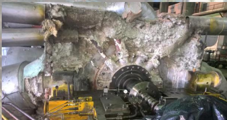
Turbine of 210 MW unit at Kota. Borescopy & UT was done
